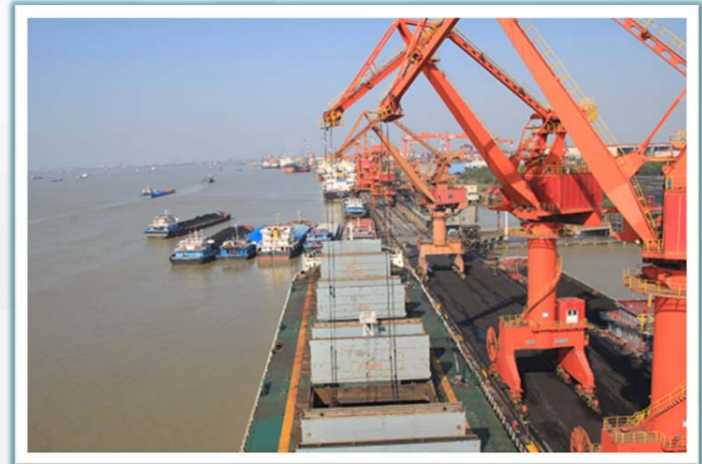
New gantry crane put into use
