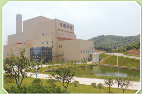
The full view of the grate furnace power generation project in Jinzhai County, Anhui Province
