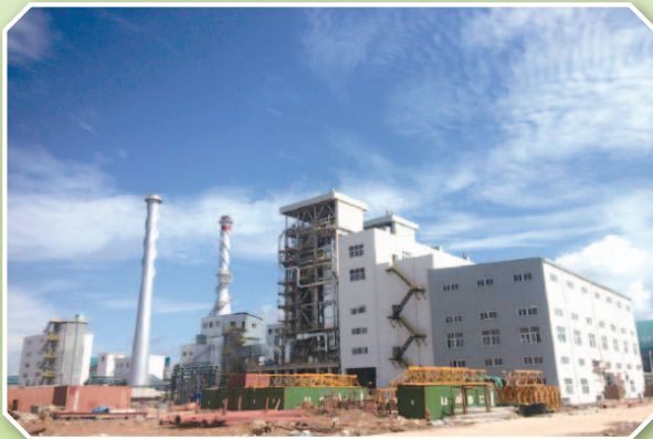
The Myanmar MCL self-owned power plants project contracted by the Group
